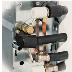
DTH2902 Valve and shut off valve
